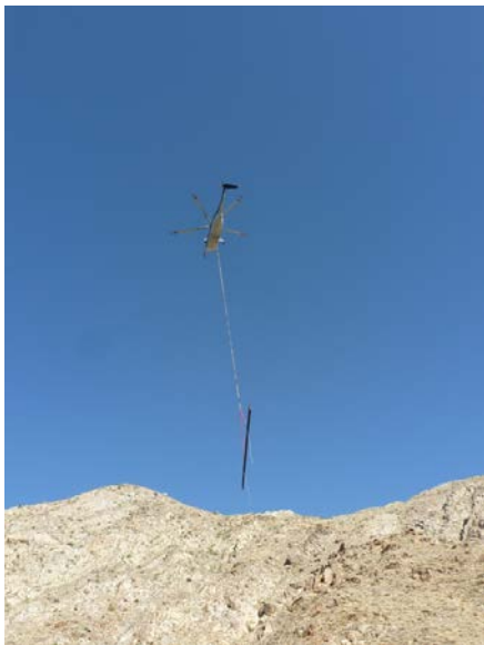
Photo 16.33 - Using Helicopters to Place Bridge Stringers on Abutments
