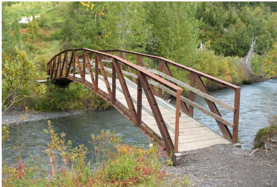
Photo 16.11 - Steel Truss Bridge
