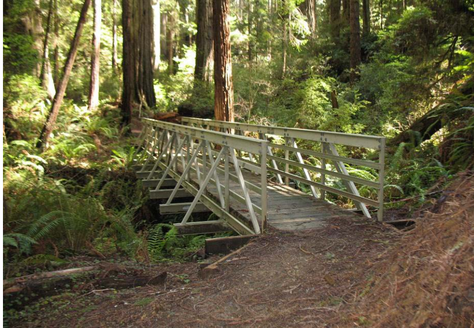
Photo 16.13 - FRP Pony Truss Bridge
