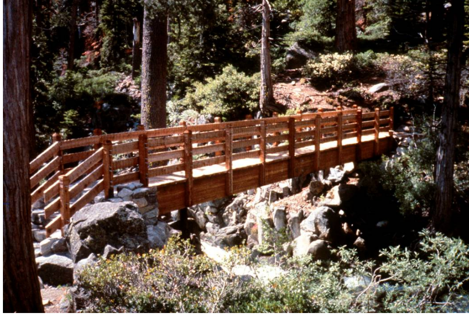
Photo 16.4 - Glulam Stringer Bridge
