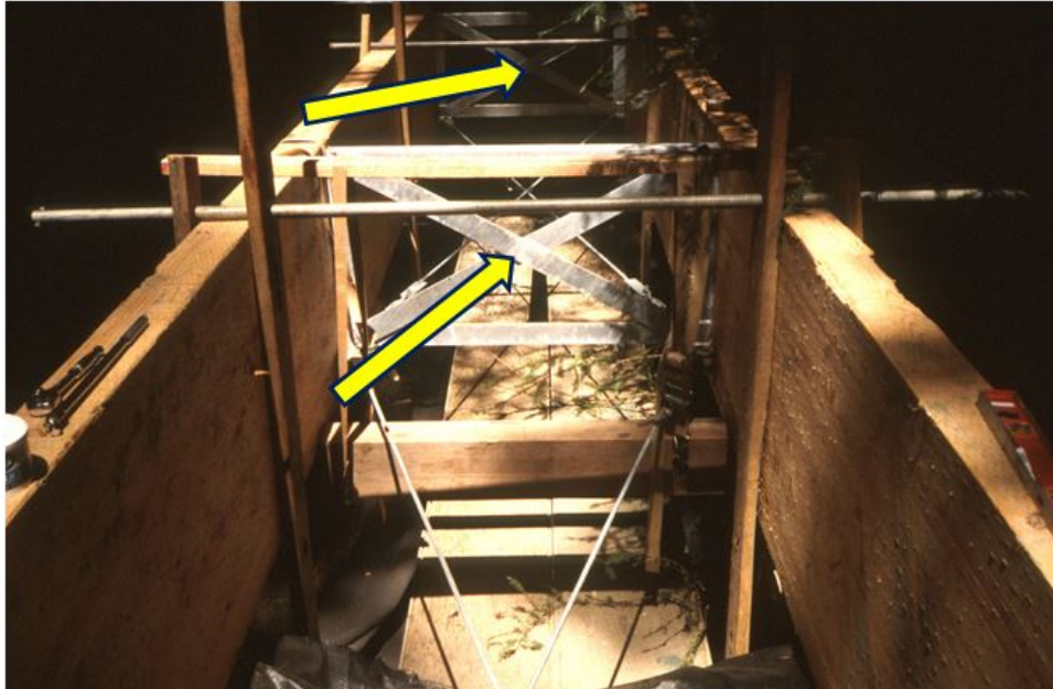
Photo 16.38 - Steel Diaphragms Between Bridge Stringers
