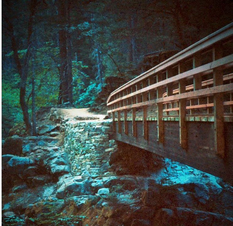
Photo 16.20 - Multi-Tier Mortared Rock Abutment
