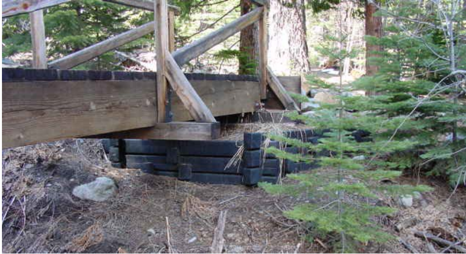
Photo 16.18 - Plastic Wood Cribbed Abutment
