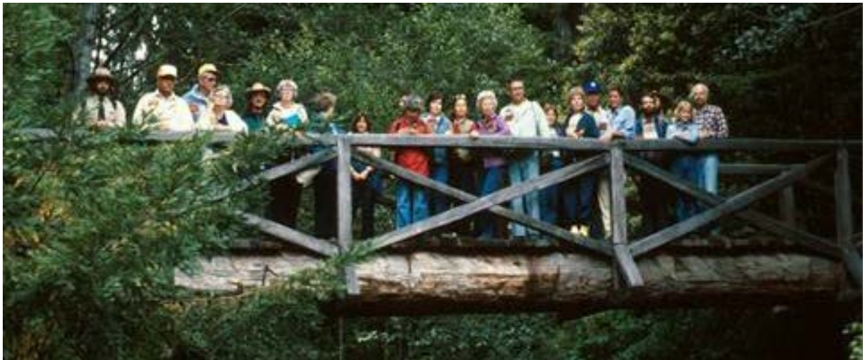
Photo 16.2 - Log Stringer Bridge
