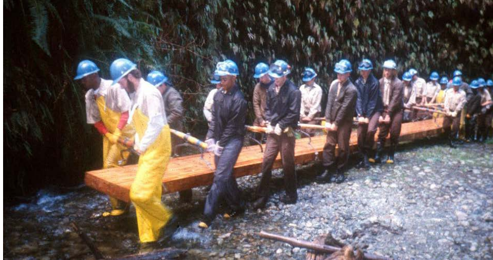
Photo 16.30 - Manually Carrying Bridge Stringers
