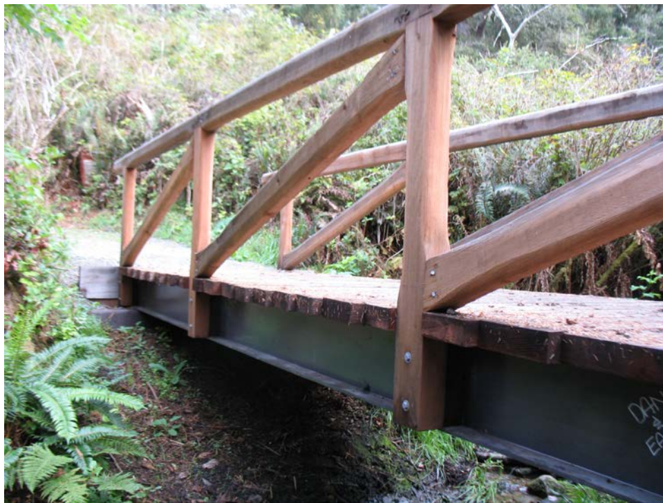
Photo 16.12 – Fiber Reinforced Plastic I Beam Bridge
