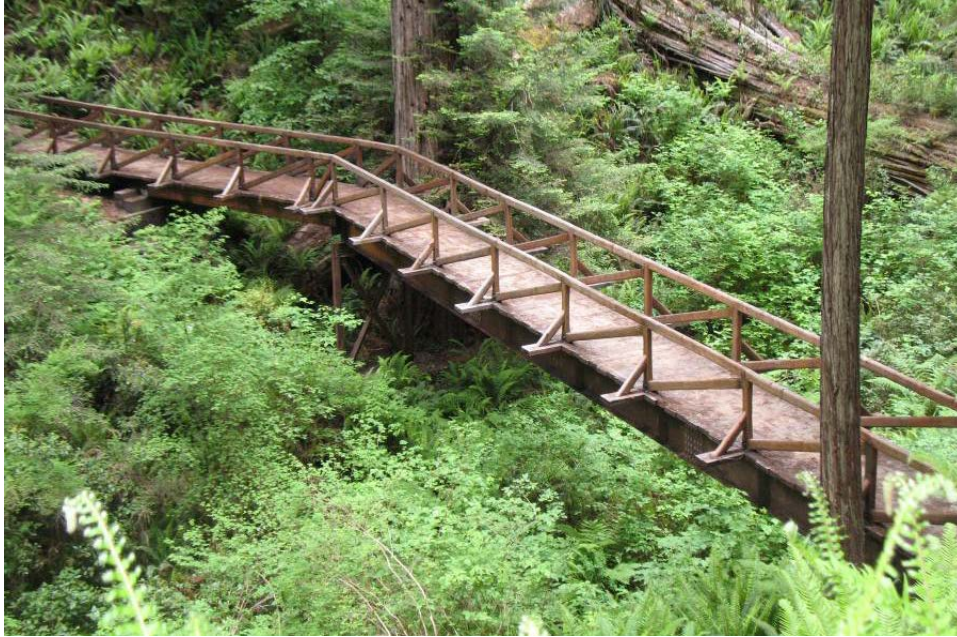
Photo 16.9 – All Weather Steel I Beam Bridge
