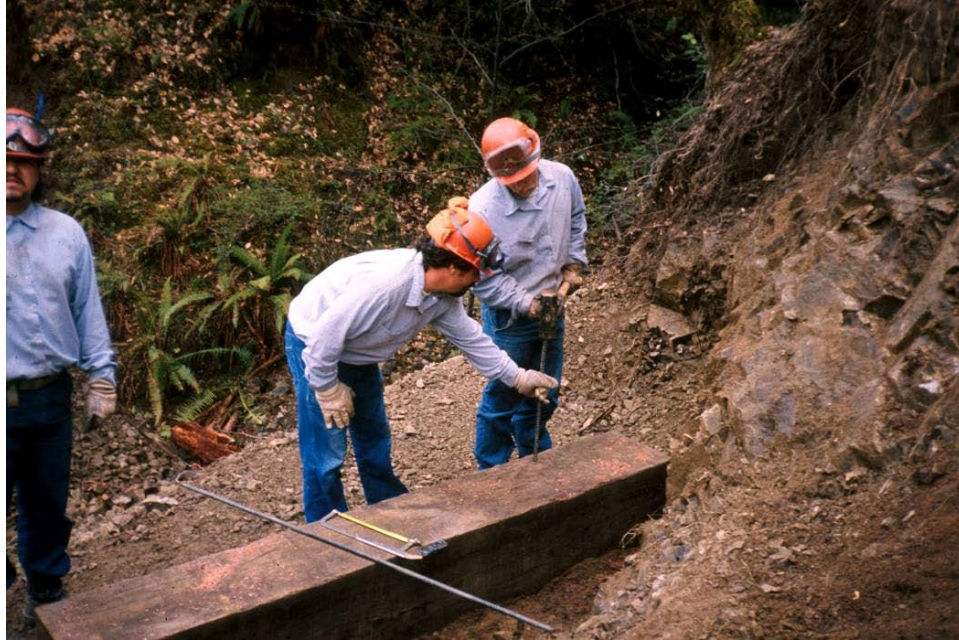
Photo 16.29 - Pinning the Mudsill With Rebar
