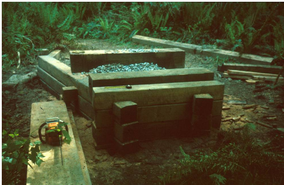
Photo 16.17 - Wooden Cribbed Abutment
