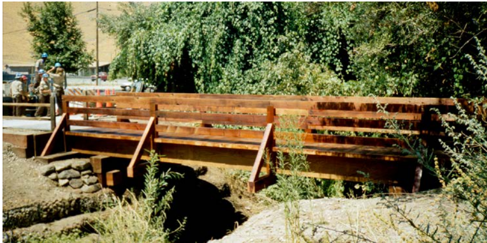
Photo 16.3 - Milled Stringer Bridge
