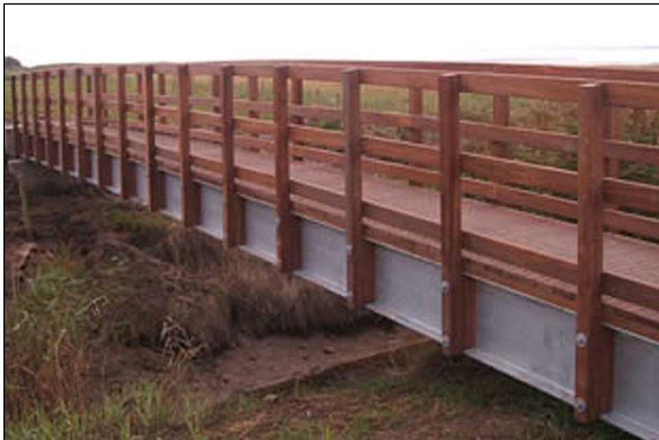
Photo 16.10 – Galvanized Steel I Beam Bridge
