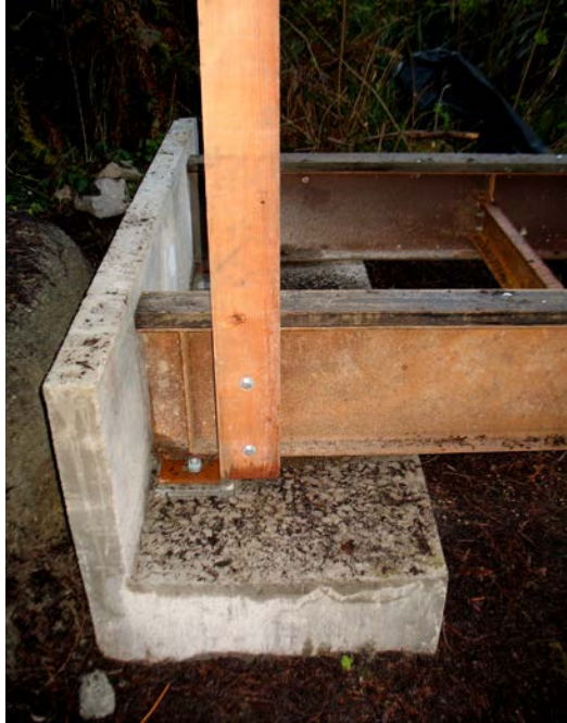
Photo 16.43 - Gussets Welded to Steel Stringers to Receive Posts
