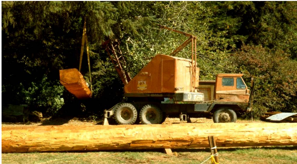
Photo 16.32 - Using a Crane to Place Bridge Stringers on Abutments
