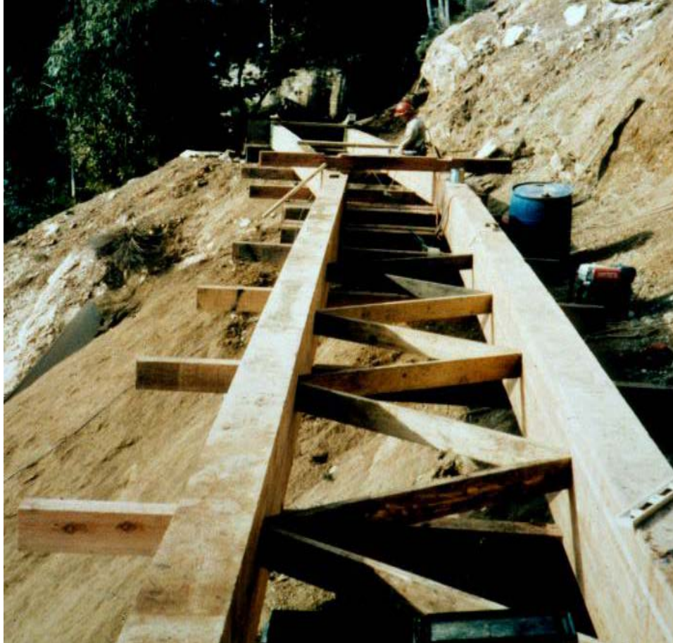
Photo 16.41 - Wooden Bridging Used to Stabilize Bridge Stringers
