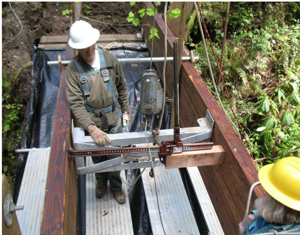
Photo 16.39 - Using High Lift Jack to Spread Bridge Stringers
