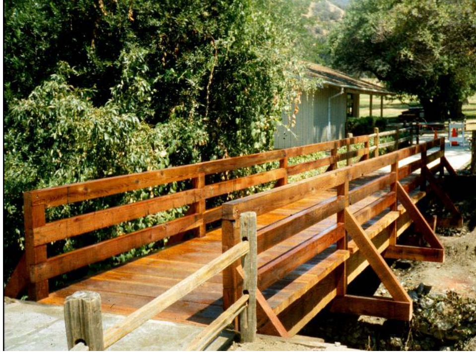
Photo 16.42 - Installed Post Sills
