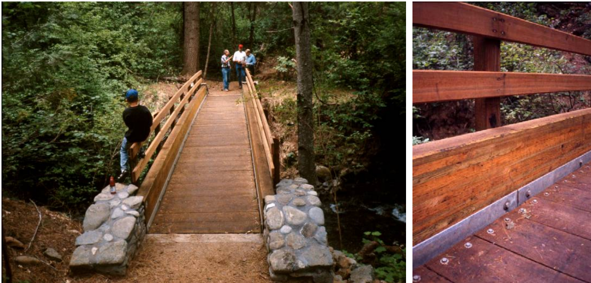
Photo 16.5 - Drop Down Deck Design
