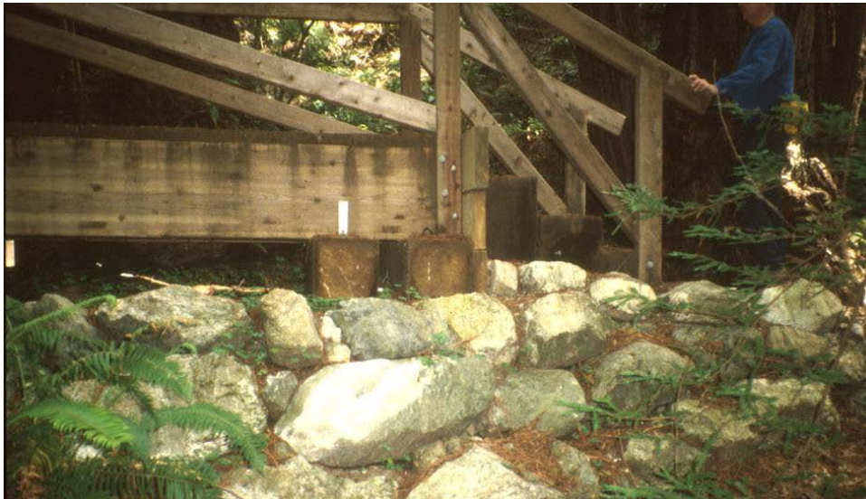
Photo 16.19 - Dry Stone Multi-Tier Rock Abutment
