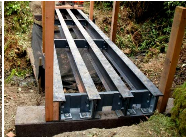
Photo 16.44 - Wooden Block Used to Bolt Post to Fiber Reinforced Plastic I Beam
