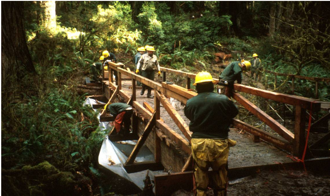
Photo 16.37 - Installing a Drop Cloth
