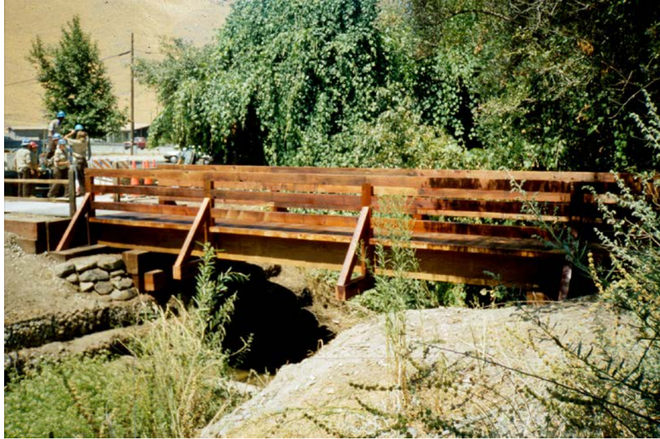
Photo 16.26 - Use of Mudsills, Post Sills, and Braces
