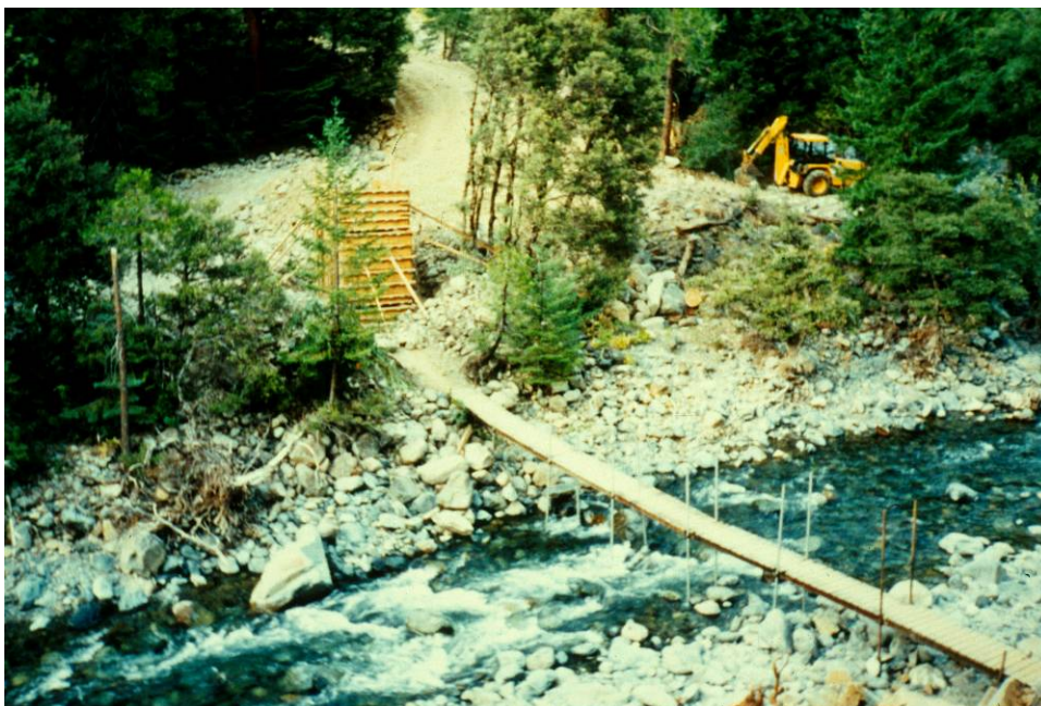
Photo 16.27 - Pipe Bridge Temporary Crossing
