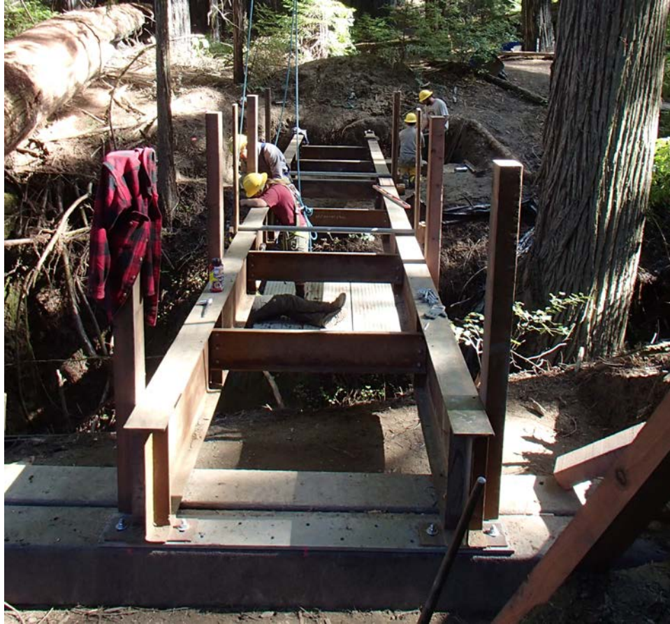
Photo 16.36 - Securing Workers to the Skyline
