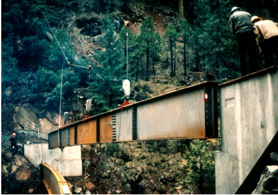
Photo 16.31 - Placing Bridge Stringers on Abutments Using Rigging
