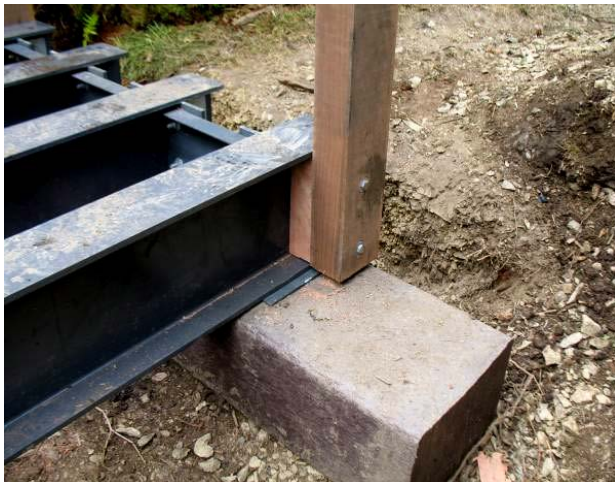
Photo 16.44 - Wooden Block Used to Bolt Post to Fiber Reinforced Plastic I Beam
