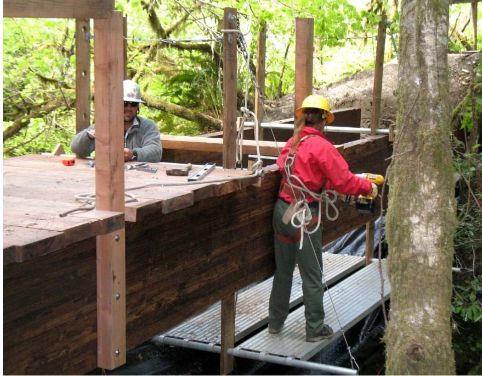
Photo 16.34 - Bridge Scaffolding Used to Assemble Bridge
