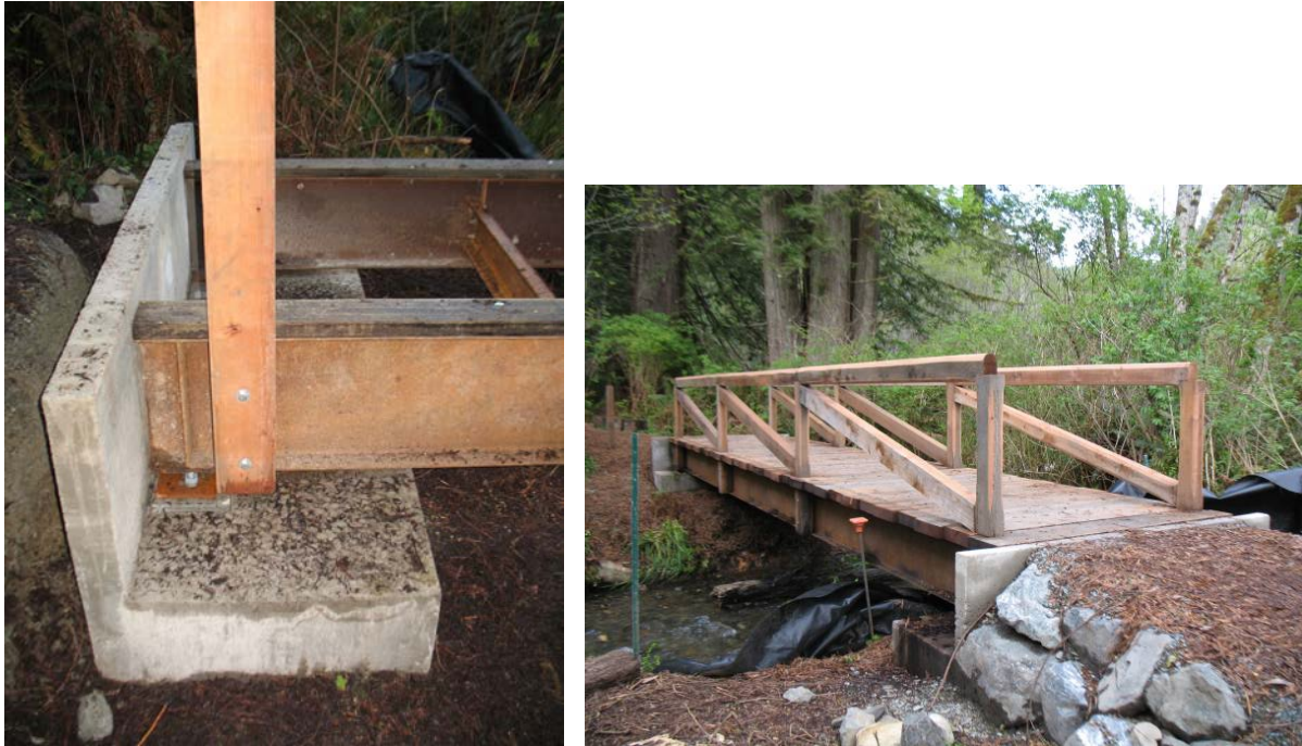
Photo 16.28 - Concrete Bridge Abutment with Stem Wall/Soil Dam
