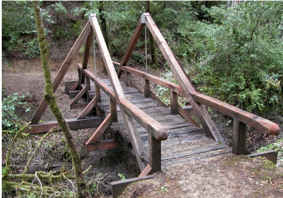
Photo 16.7 - Overhead Wooden Truss Bridge Design
