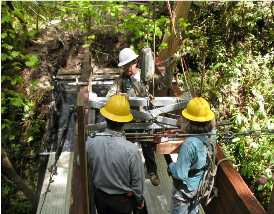
Photo 16.35 - Using Skyline, Blocks, and Hoist to Move Loads
