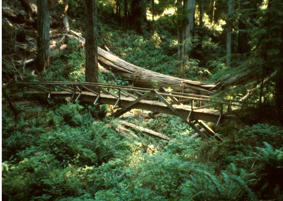
Photo 16.8 - Hip Truss Bridge Design
