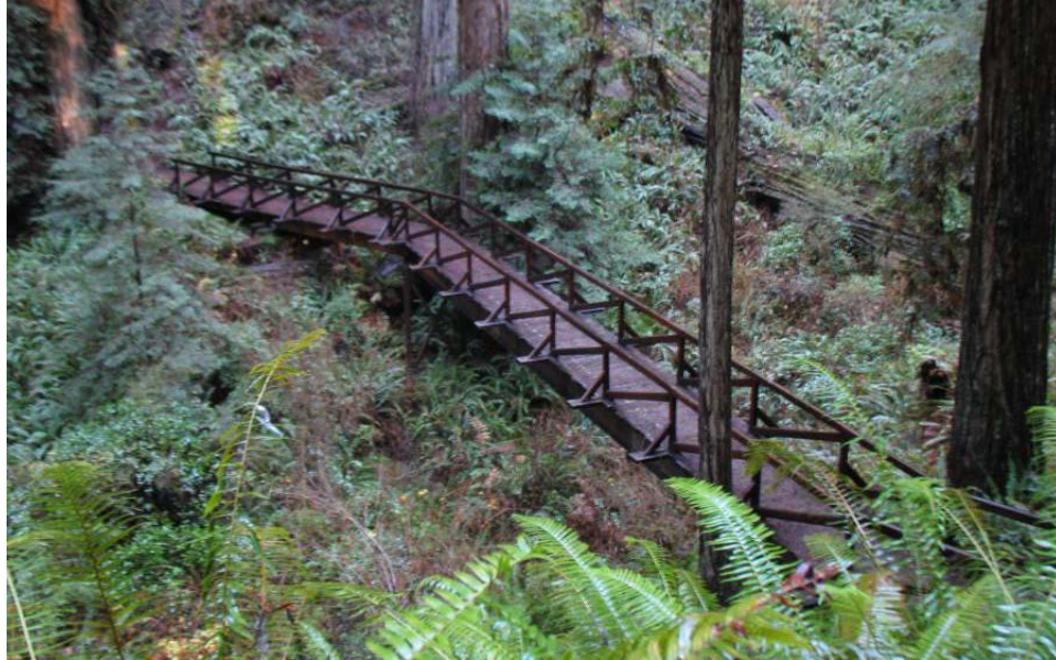
Photo 16.24 - Using Trestle to Alter Bridge Alignment
